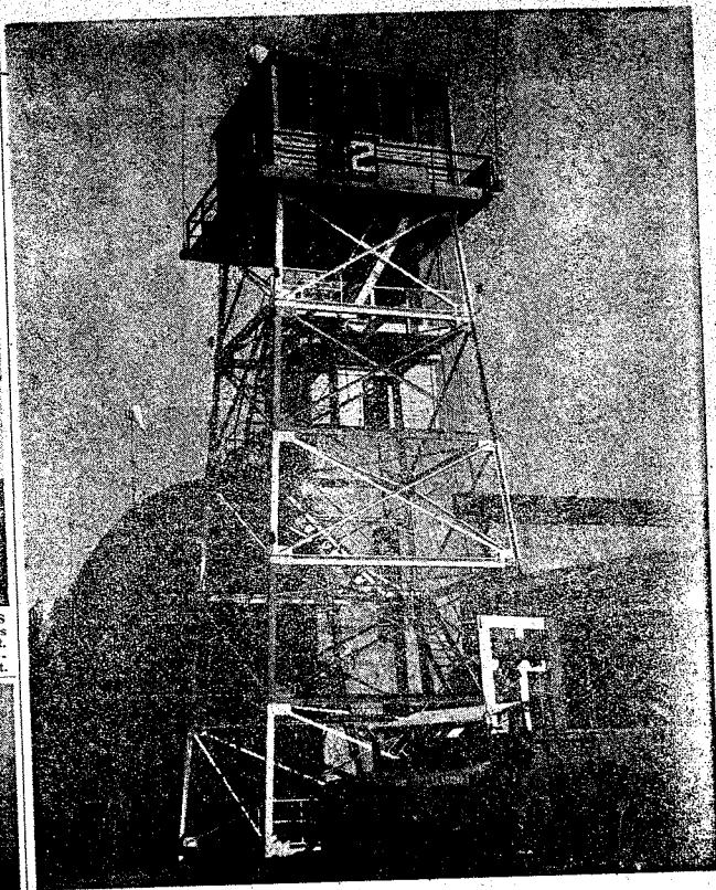
GUIDING HAND —The control tower is the center of activity at Lawson field. From the tower, landing and take-off instructions are issued to aircraft along with altimeter readings, weather reports, and other messages necessary to safeguard pilots, their crew, and the aircraft.
