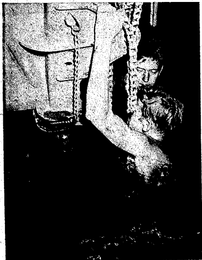
THEY ARE NOT SWIMMING —The 78th Engineers enjoyed their underwater work in Florida, but suggest that no one attempt to construct a bridge in Alaska. In this picture Pfc. William Haines, foreground, and Pfc. Walter Howell place a locking pin on the adjustable transom.
