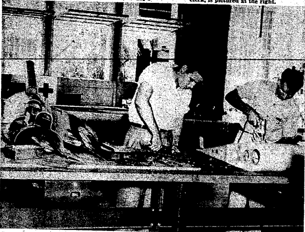
SHEET METAL WORKERS —J. K. Barlar, left, and A. B. Williamson, aircraft sheet metal workers, repair the accessory cowling and control surface of a horizontal stabilizer section.
